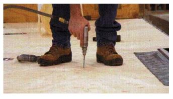
5/8" TONGUE AND GROOVE, MARINE GRADE PLYWOOD FLOOR
