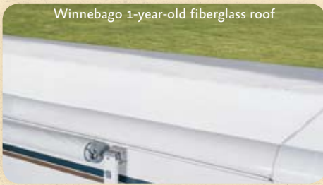
Winnebago 1-year-old fiberglass roof
