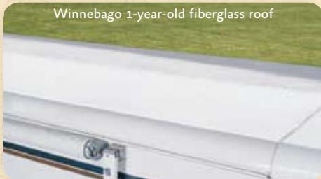
Winnebago 1-year-old fiberglass roof
