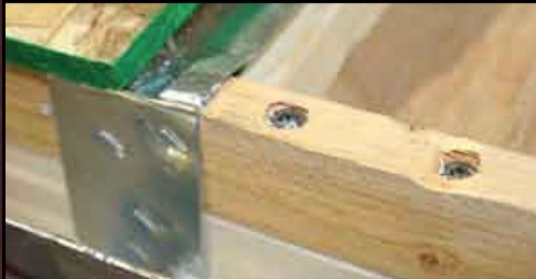
Our construction methods using screws and additional hurricane style strapping creates a unibody out of the floor, sidewalls and roof. This insures a tight fitting, long lasting, strong structure for years of use and enjoyment.
