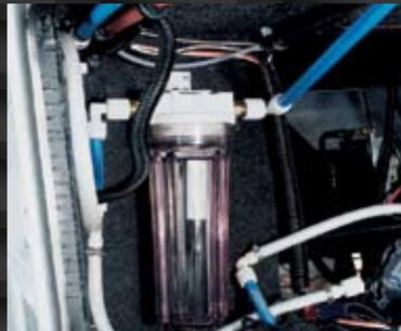
The water filtration system provides safe clean drinking water through all the water lines and water heater.
