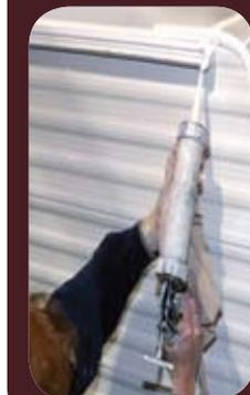
A secondary "cap seal" is applied over all exterior corner joints. The "cap seal" is a non silicone base sealant that will not blacken or yellow with time.
