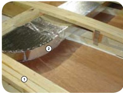
Our roofs are 4 1/2" solid wood bow truss rafters. Designed for good drainage and maximum strength. Features include:
