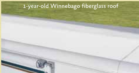
1-year-old Winnebago fiberglass roof
