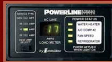
**WEB POWERLINE®** This energy management system monitors electrical usage and automatically cycles appliances on and off to prevent tripped campground circuit breakers.
