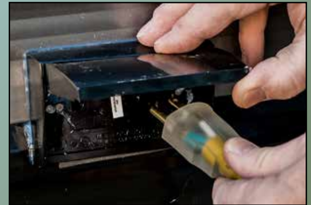
Convenient Outside GFCI Protected and Covered Outlet.
