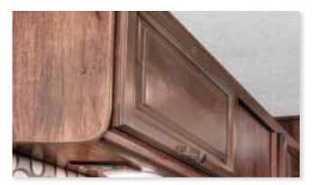
The Reactor features raised panel cabinets that are screwed and glued—never stapled.
