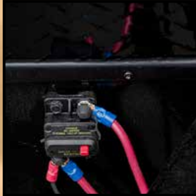
12V MAIN BREAKER / BATTERY DISCONNECT
