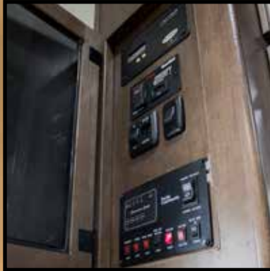
CENTRAL CONTROL PANEL
