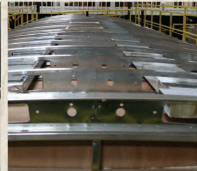
Walkable steel truss roof system
