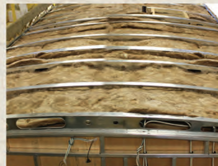
Steel truss roof system
