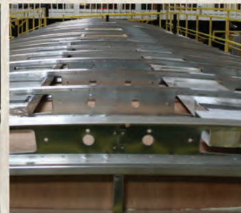
Walkable steel truss roof system
