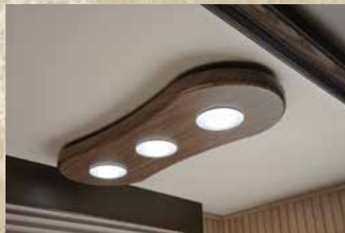
LED interior lighting provides: • 80% less power • Emits less heat • LED's last 30,000 hours vs. 1,000 hours of halogen
