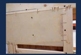
Every Northstar is screwed together at every single joint. Cabinets screwed in from the outside through the wall and also screwed together on the inside. Exterior plywood and low fomelhyde emmission paneling make for superior strength & breathability. Northstars are made to last a long time and endure many miles and off road use. It's the Northstar way!
