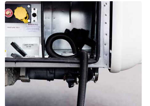
Macerator Sewage Discharge With Manual Disconnect
