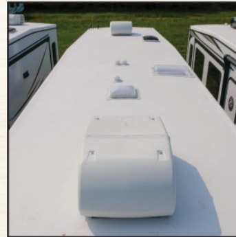
PVC ROOF MATERIAL WITH VENTED ROOF DESIGN AND SOLAR PANEL
