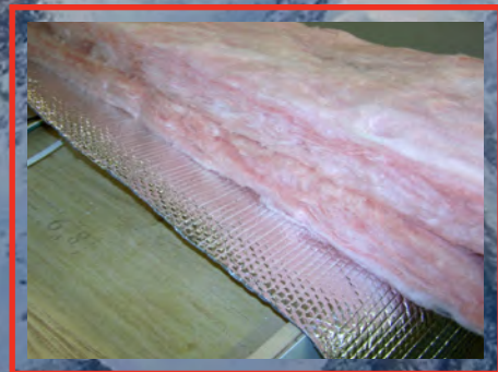
Triple Layered Four Seasons Roof Insulation
