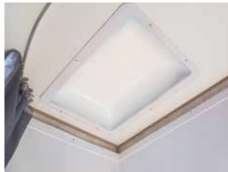
Skylight over Tub
