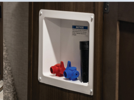
Washer/Dryer Prep Ready to add a combo washer/dryer unit.
