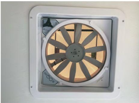
High Output Attic Fan in Bathroom
