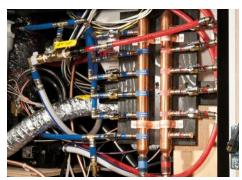
A copper water manifold comes standard, ensuring equal water pressure throughout your home. And each water line is clearly labeled and has its own shut-off valve, allowing you to isolate a single line without shutting off water to the rest of your home.
