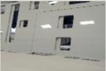
Vacuum Bonded Walls with Azdel.
