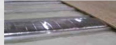
3" Aluminum floor studs, heat duct and 5/8" tongue and groove plywood floor.
