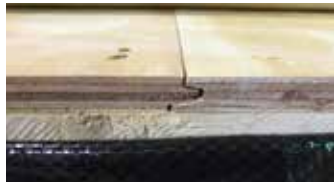
Tongue & Groove Plywood Flooring
