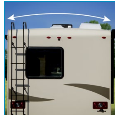
TPO Crowned Roof for Easy Water Runoff
