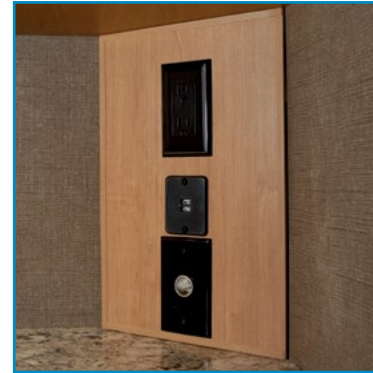
Bedroom Charging Station and Dedicated CPAP Outlet and Storage Location
