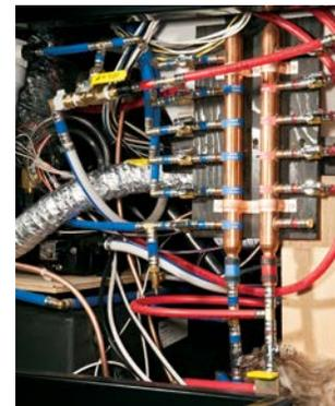
A copper water manifold comes standard, ensuring equal water pressure throughout your home. And each water line is clearly labeled and has its own shut-off valve, allowing you to isolate a single line without shutting off water to the rest of your home.
