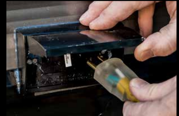
Convenient Outside GFCI Protected and Covered Outlet.
