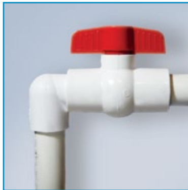
1" Fresh Water Tank Drain
