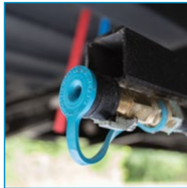
Exterior LP Connection
