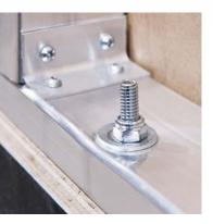
Residentially-hung sidewalls are carriagebolted into the floor for solid construction and superior strength.
