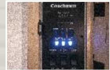
Centralized Control Panel indicates tanks, battery levels and operating components.
