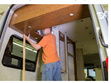
end gables and upper cabinets are all screwed together and fastened with steel angle brackets for superior strength and quality. Cabinets are anchored into the coach sub-floor and wall blocking that is adhered to the inside wall to ensure their strength. This extra step adds stability to the cabinetry and it also helps to ensure a more peaceful, rattle-free ride!
