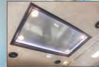
Backlit Coffered Ceiling w/LEDs
