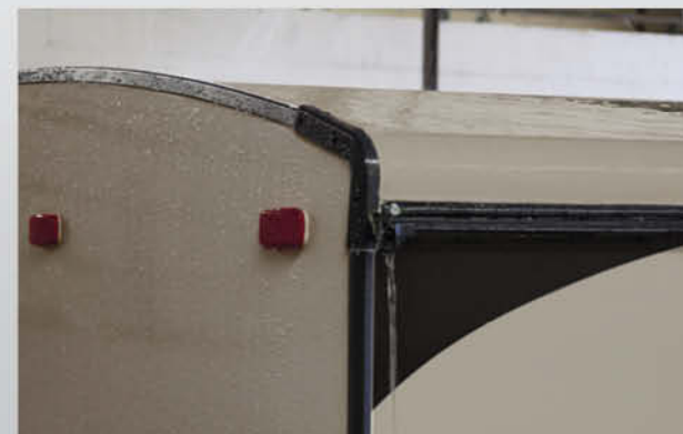
TPO Roll Over Roof
