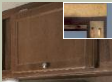
Screwed lumbercore cabinetry with hardwood mortise and tenon doors
