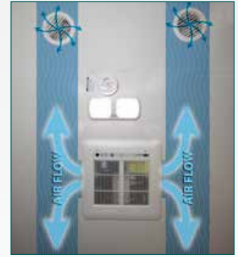
The H-ducted A/C distributes the cool air evenly throughout the travel trailer.
