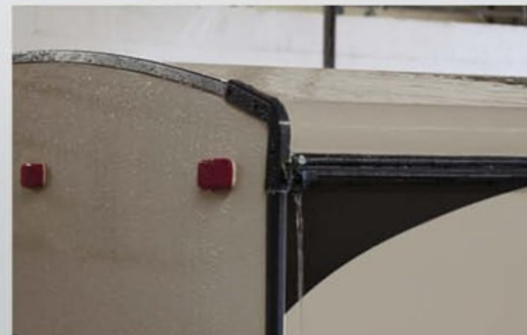
TPO Roll Over Roof
