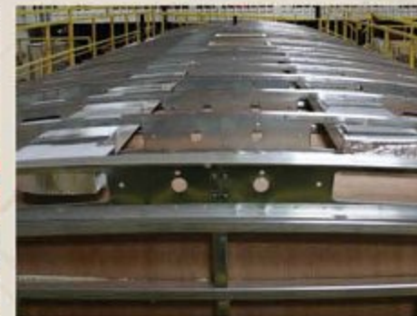
Walkable steel truss roof system
