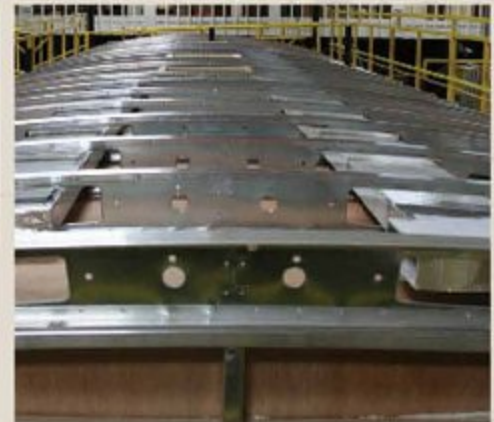
Walkable steel truss roof system
