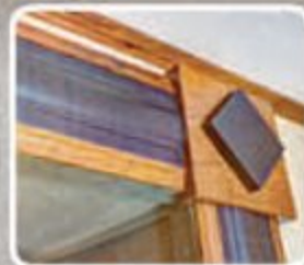
CROWN MOLDING IN LIVING ROOM
