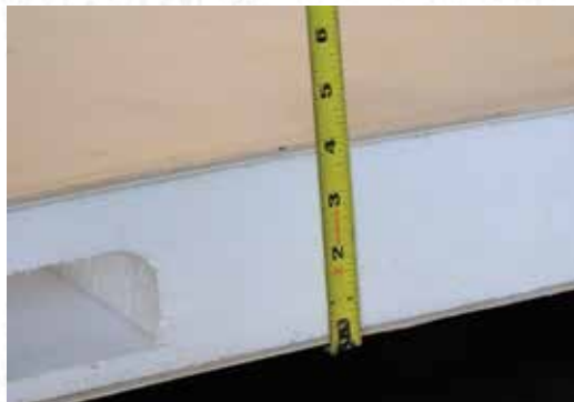
4" thick roof with built-in insulated A/C ducts.
