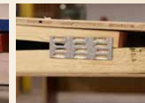
THEM They use smaller and only on one side of truss.
