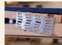
US We use large oversized nail plates on both sides.
