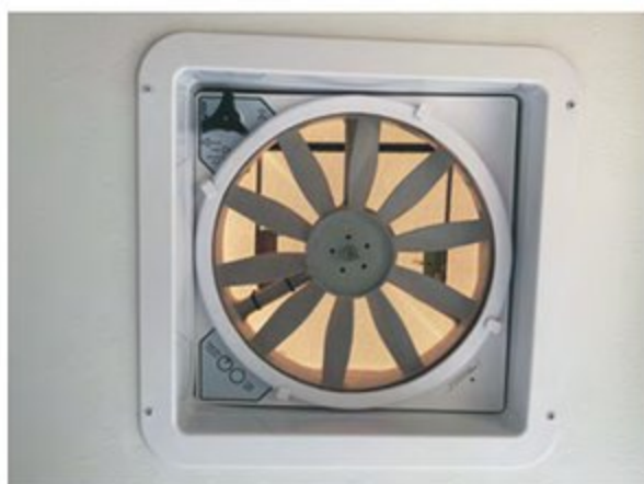
High Output Attic Fan in Bathroom
