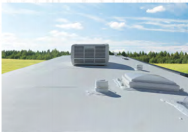
Seamless Roofing Membrane with Heat Reflectivity
