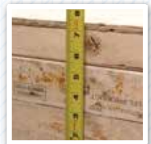
7" HEADER BEAM VS. 2" X 6" LUMBER
