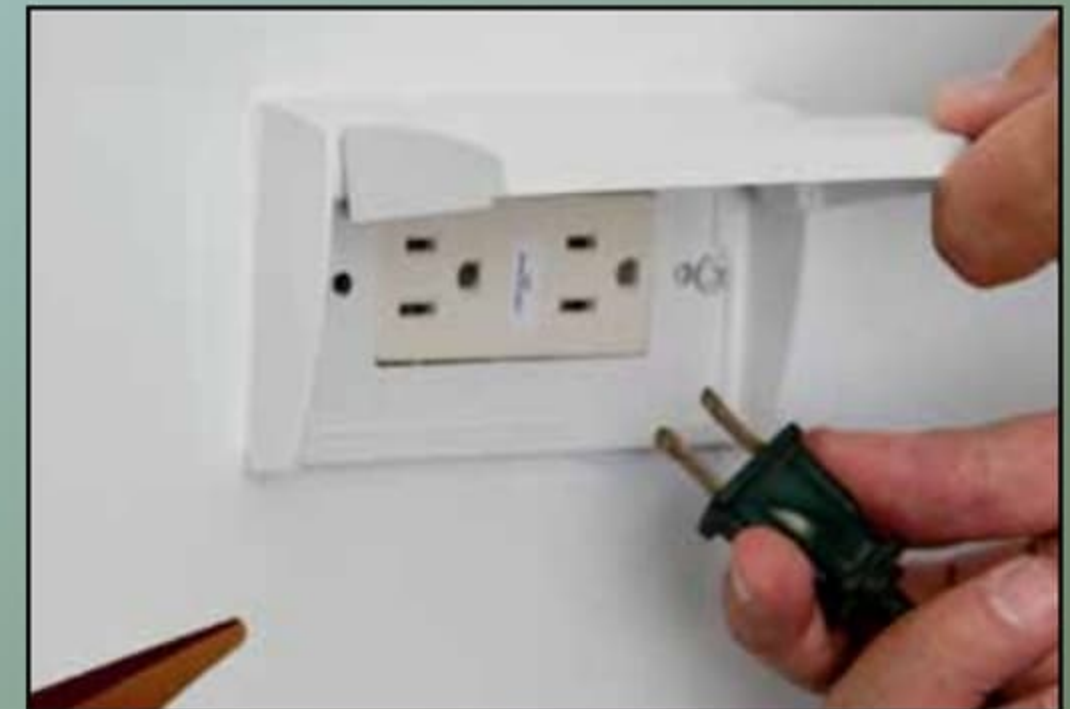
Convenient Outside GFCI Protected and Covered Outlet.
