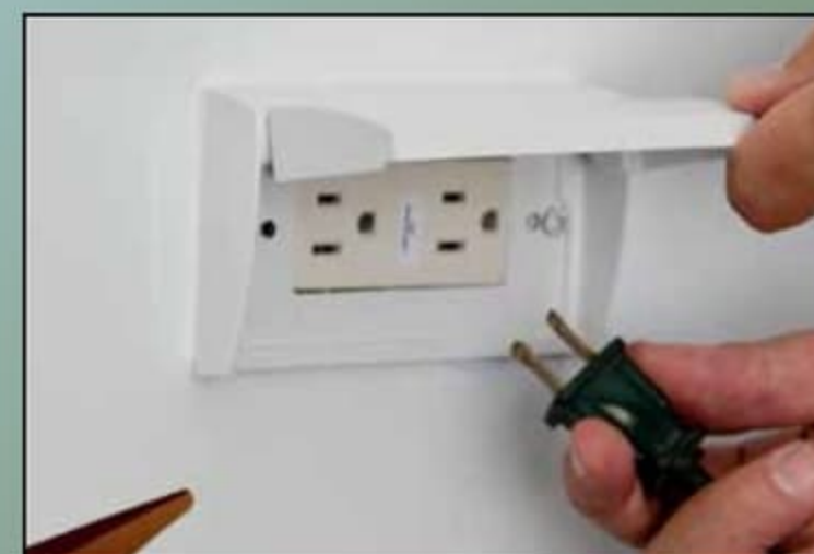
Convenient Outside GFCI Protected and Covered Outlet.
