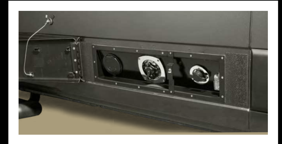
2 Water hookups are concealed behind a natural design.
