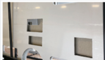
TALON GEL COAT GLASS FUSED FIBERGLASS WITH COMPOSITE BACKER
