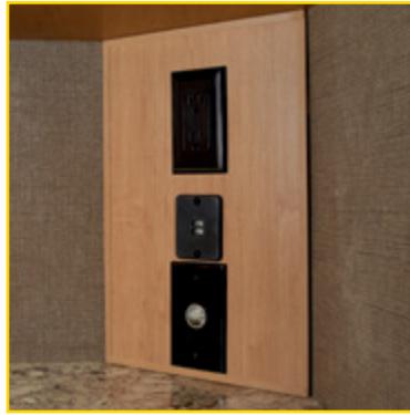
Bedroom Charging Station with Dedicated CPAP Outlet and Storage Location
