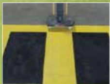
Weight Scales Recessed In the Floor
