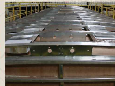
Walkable steel truss roof system
