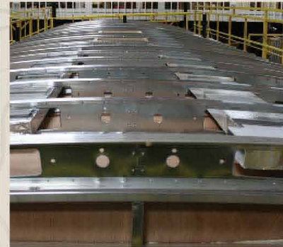
Walkable steel truss roof system
