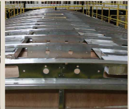
Walkable steel truss roof system
